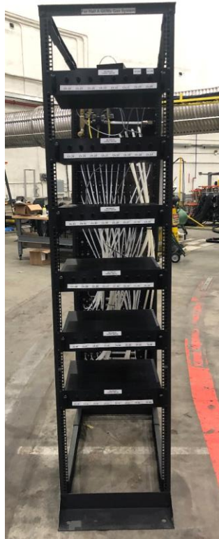
Rear view of SBS gas distribution panel in Hall A
